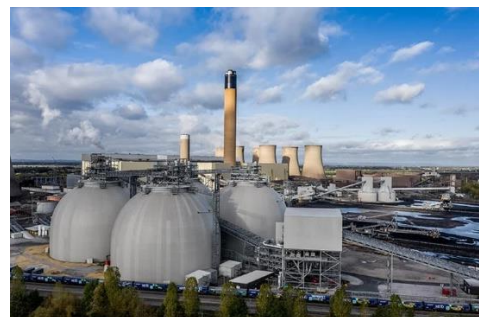
Biomass Power Plant
